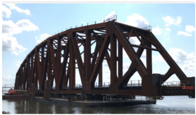
New Terminal Merchants Bridge – Venice, Illinois 2021
